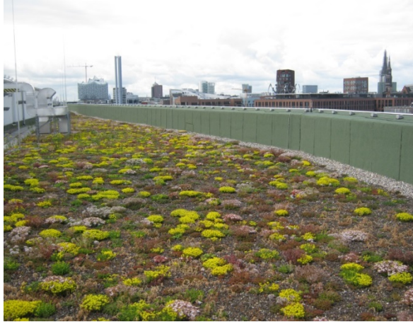
Fig. 2 View over the HCU green roof
