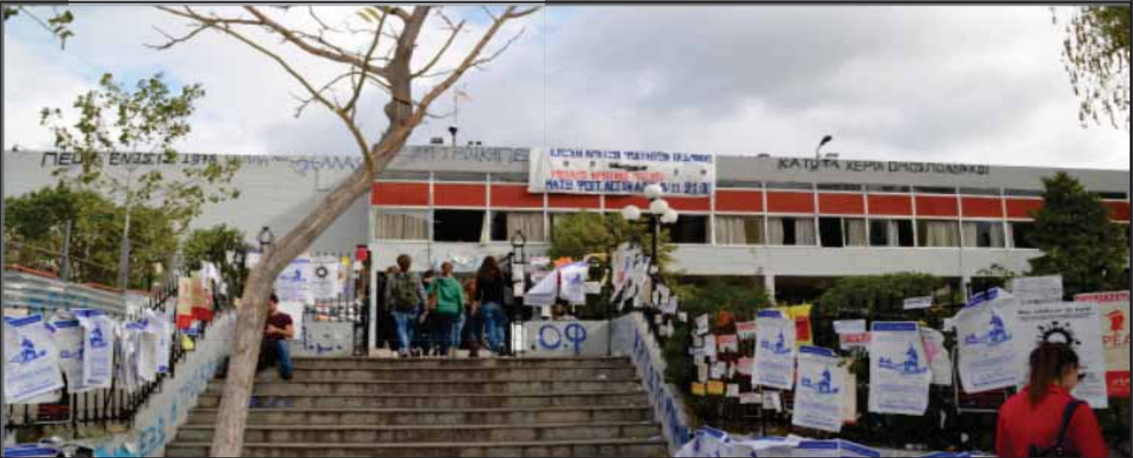
7.1 AUTH Cafeteria building entrance (Own compilation, 2013)
