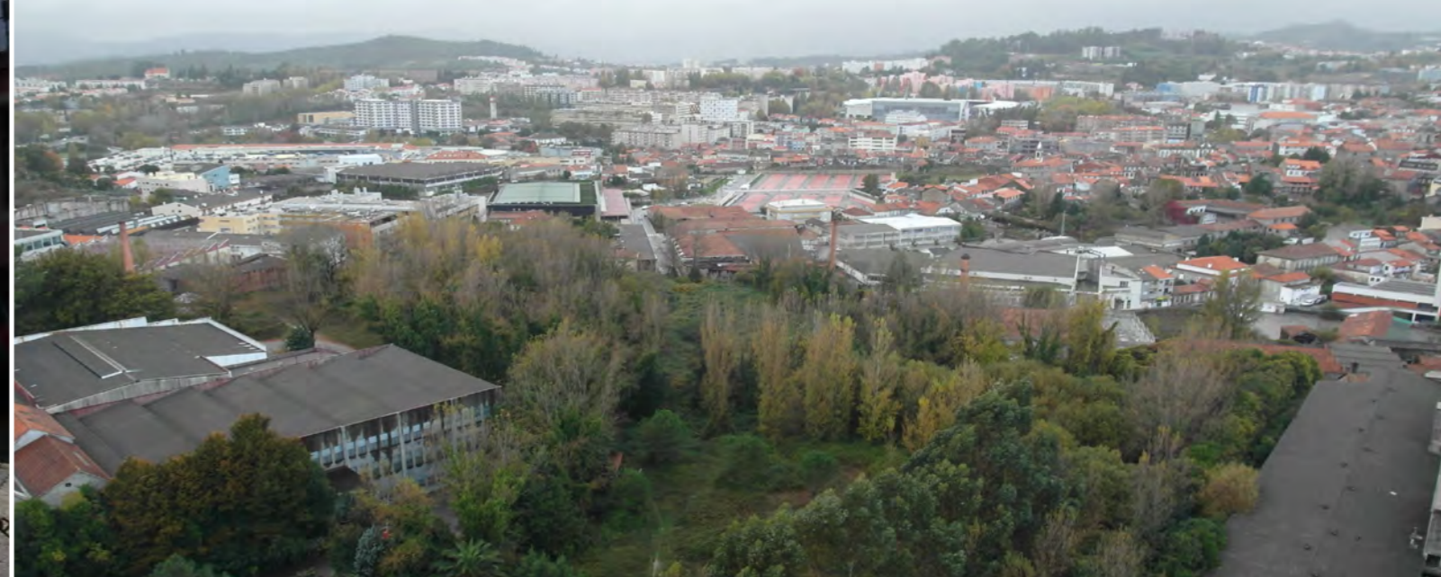
3.8: AERIAL VIEW OF SITE SHOWING BUILDING D ROOF
