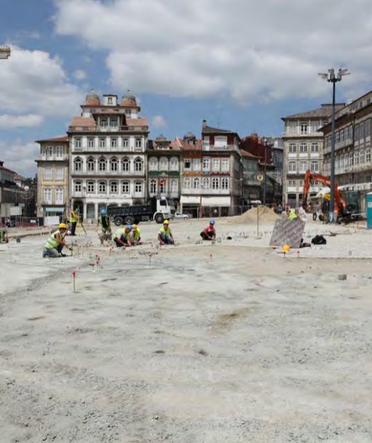
F.1: CONSTRUCTION IN GUIMARAES TOWN SQUARE
