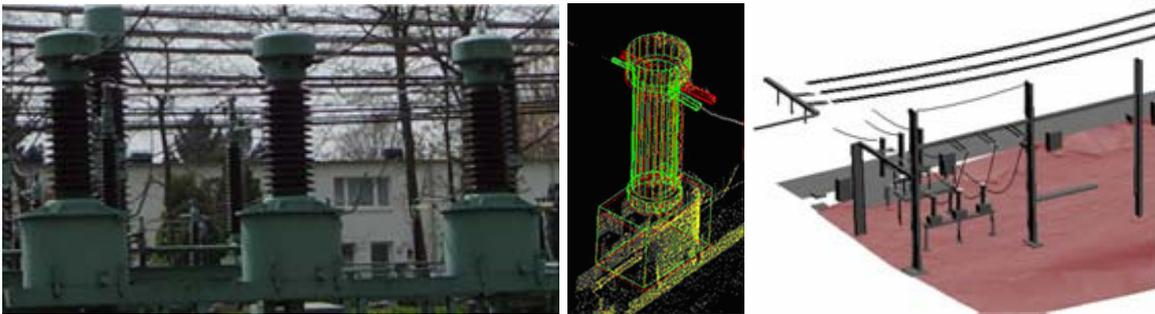
Fig. 3: Isolators (photo left) constructed in Cyclone including a superimposed copy (centre), part of the 3D model (transformer station), constructed in 3Dipsos from Trimble GS101 data (right)
