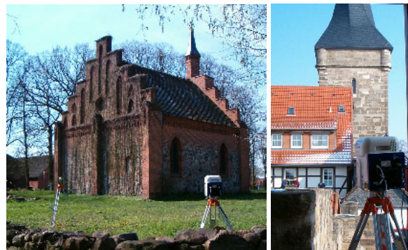
Figure 5: Terrestrial 3D laser scanning system Mensi GS100 in use: church Raduhn (left) and West Tower (right)
