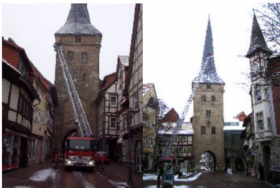
Figure 4: Mobile turning ladder at the West Tower in Duderstadt for signalling of control points and for image recording
