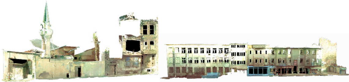
Figure 3. Coloured point cloud of building facades in the Historic Peninsula
