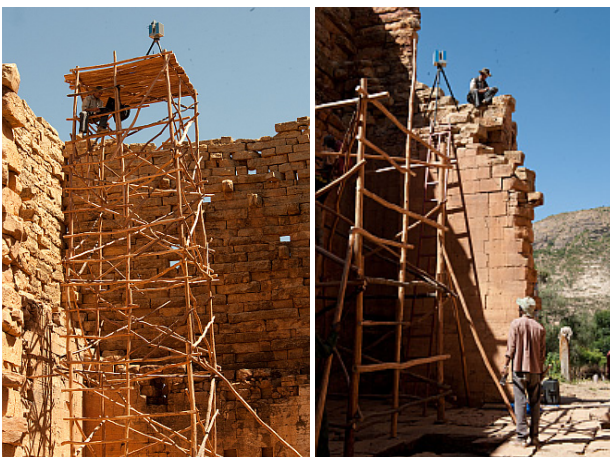
Figure 2: Scanning on scaffolding (left) and on top of the wall (right) using the IMAGER 5006 from Zoller + Fröhlich
